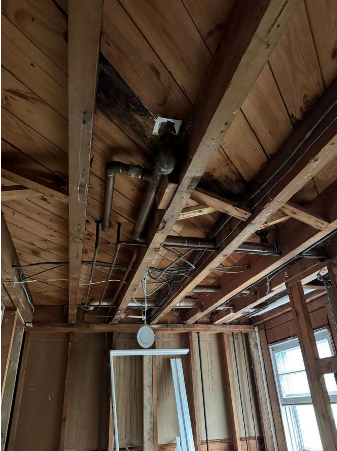
Before: the old copper and cast-iron drain lines
